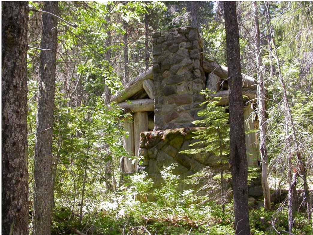
Figure 6. Cooper Spur warming shelter from east.
