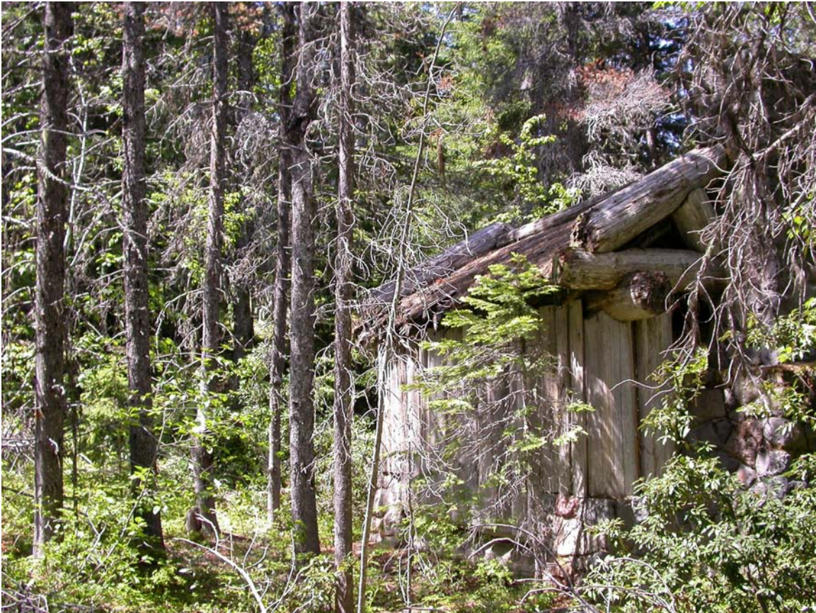
Figure 7. Cooper Spur warming shelter from west.
