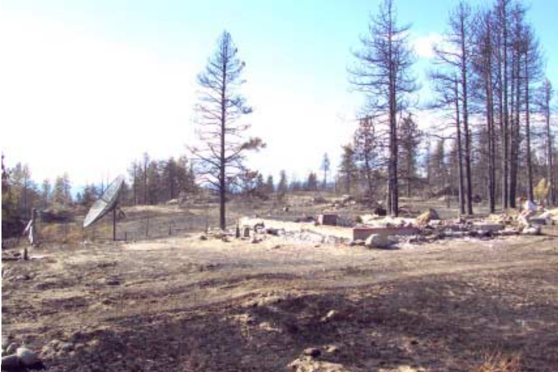
A house burned in the Virginia Lake fire. Note that the house is in an open, sparsely vegetated area. Photo by Peter Morrison, August 23, 2001.
